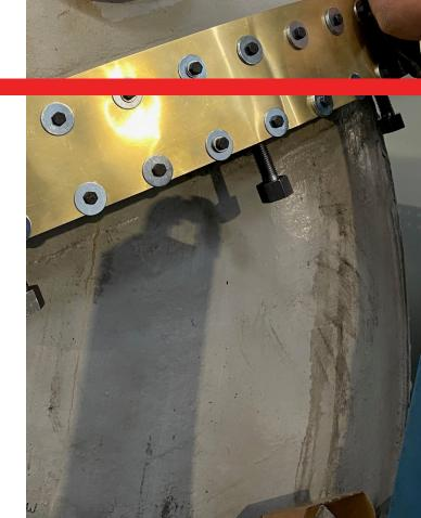
Once the mold was set in place Belzona Belzona 7111 (Marine Grade) was mixed and then poured into the mold. Once the Belzona 7111 (Marine Grade) was fully cured, the mold was removed and the sharp edges were sanded.
